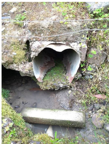
Figure 5: Photograph of the number 53 culvert entrance (taken 21 November 2020).
