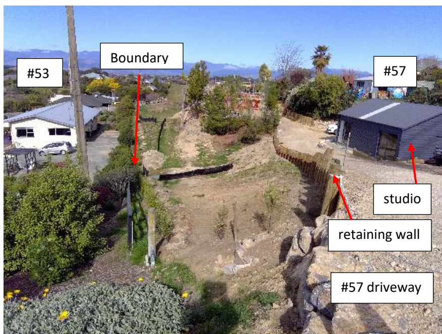
Figure 1: Photograph of retaining wall and driveway (taken 11 August 2020).
