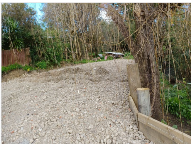
Figure 2: The area behind the retaining wall
