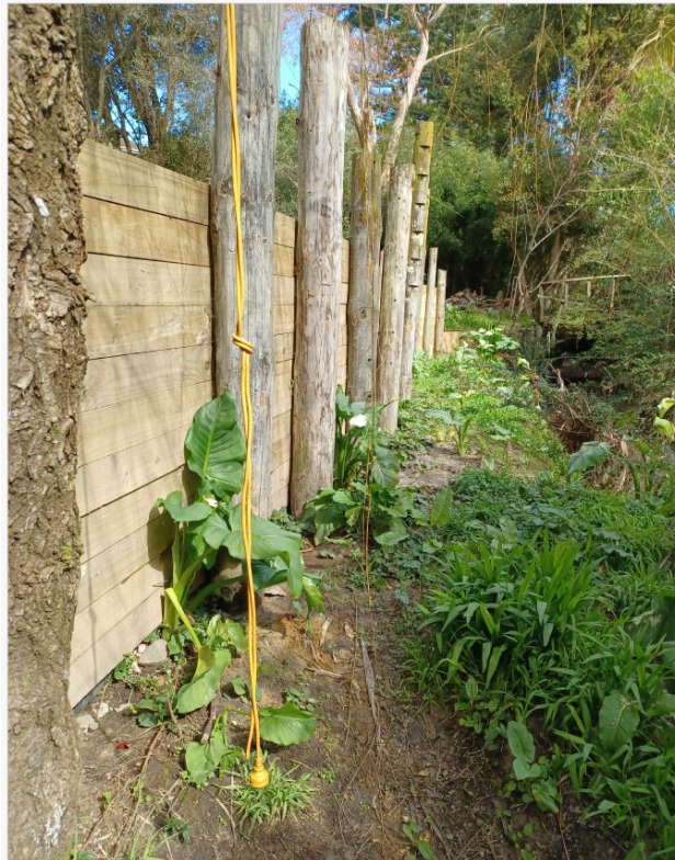
Figure 1: The retaining wall under consideration
