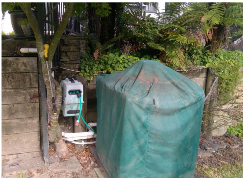
Figure 3: View of the retaining wall, tank, hose reel and pipes.
