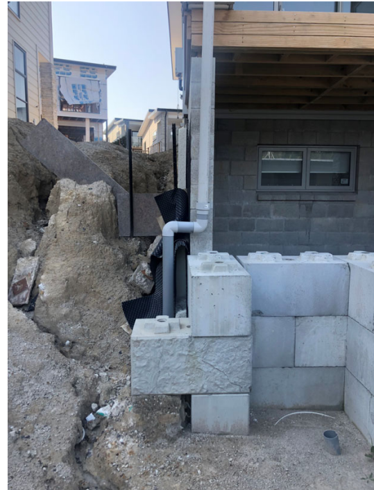
(b) Sloping ground to rear of wing wall
