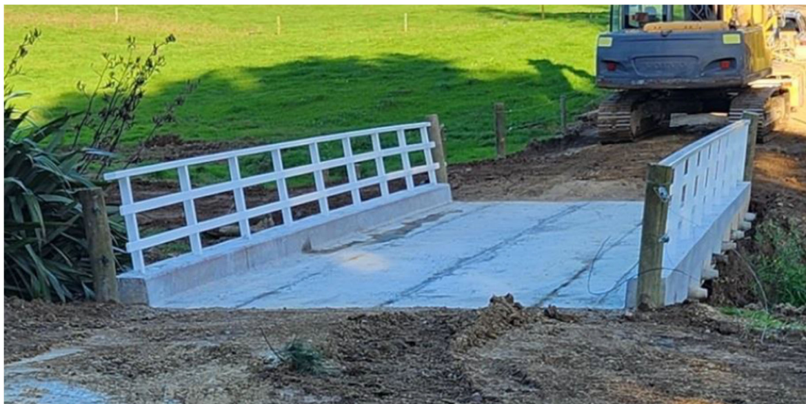
Figure 1: View of bridge looking south 1
