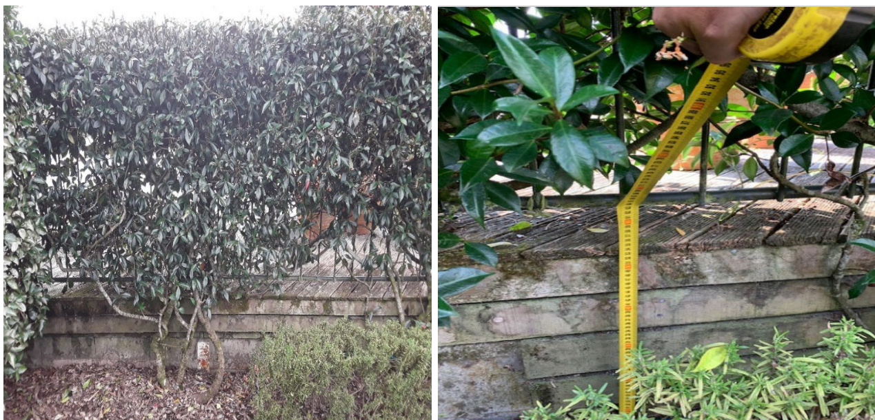
Figures 3 (left) & 4 (right): Photographs of the southern section of the barrier, showing the deck, metal fence and the hedge.
