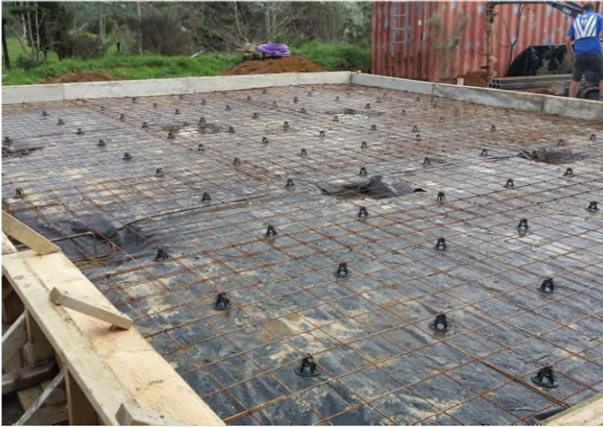
Figure 1: Photograph of formwork, reinforcing steel, and vapour barrier
