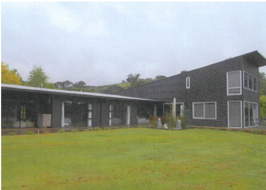
Figure 1: External view of the dwelling
