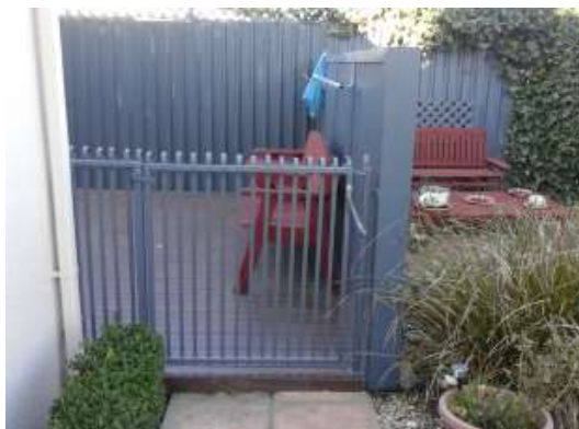
Figure 2: south fence & south gate (looking from the rear yard)
