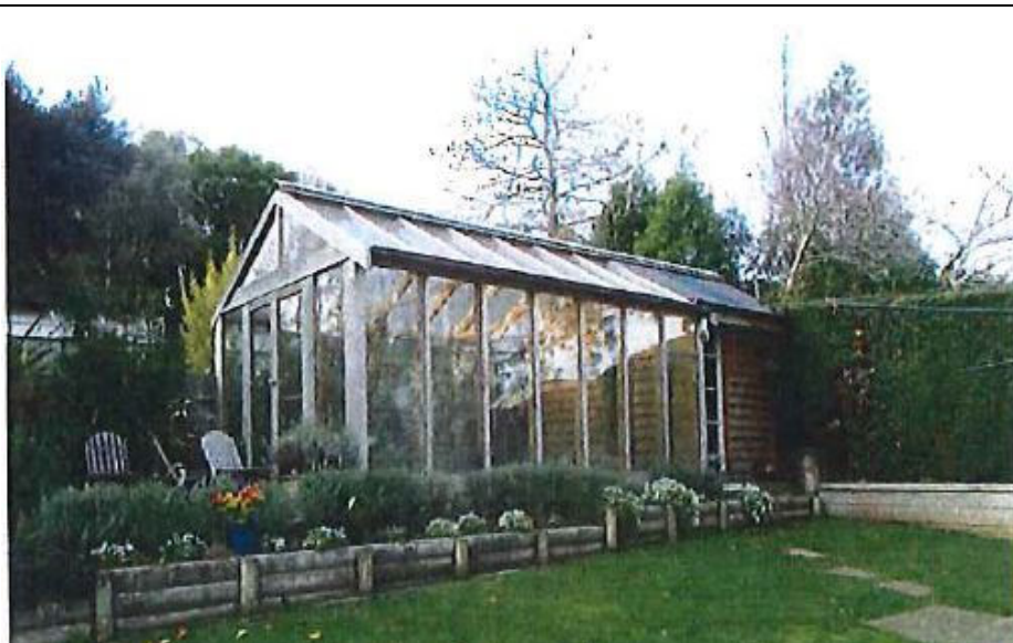
Figure 1: Photograph of the outbuilding
