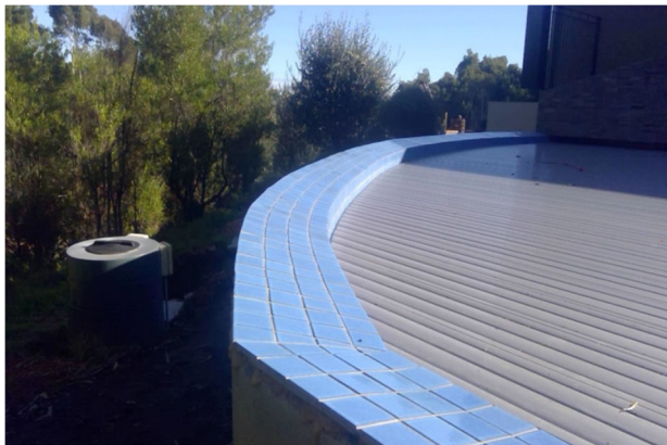
Figure 2 (above): top of the masonry pool wall
