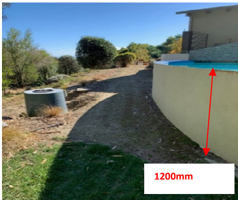
Figure 3 (above): masonry pool wall & wastewater treatment tank
