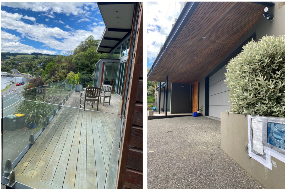
(a) Top view of deck
