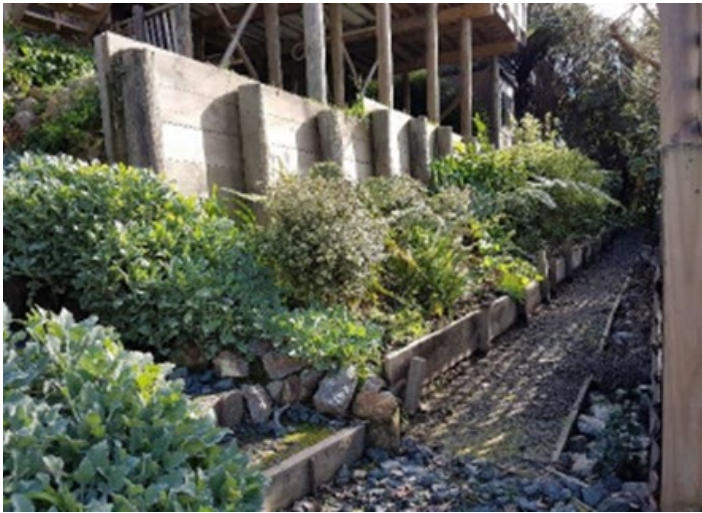
(a) The retaining wall shown below the new deck
