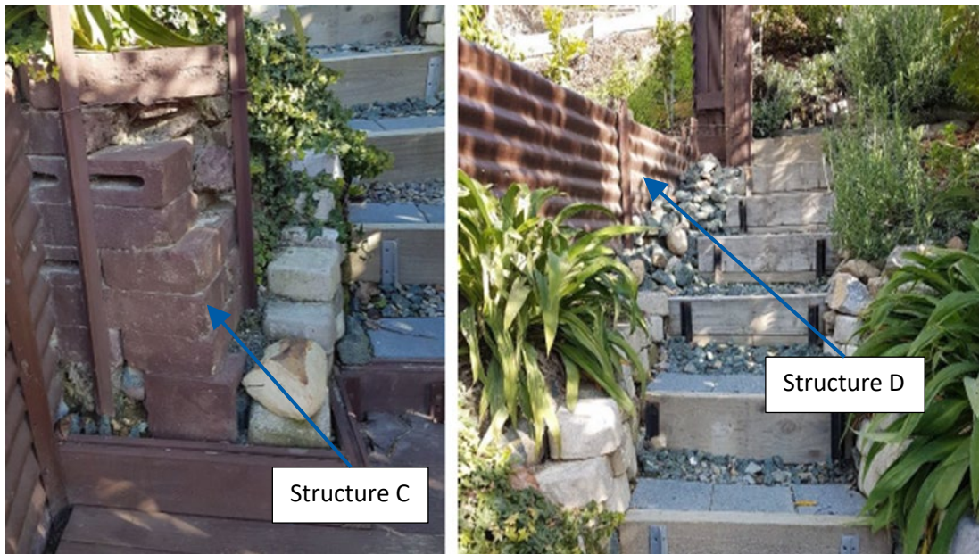
(b) Dry-stacked masonry (structure C) (c) Corrugated iron fencing (structure D)
