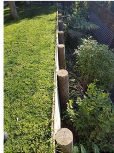
(b) Top of the retaining wall
