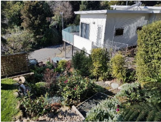
(c) End of retaining wall
