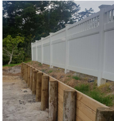
Figure 1: Photograph of existing boundary fence from the proposed pool side
