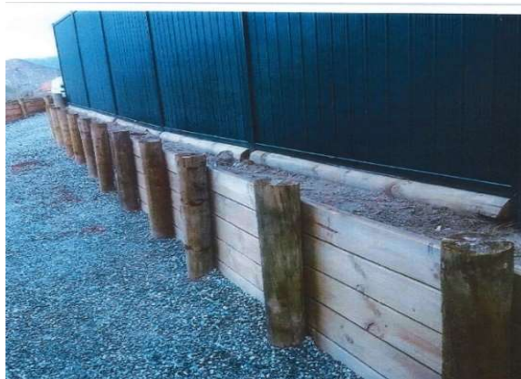
Figure 1: Photograph of Part 1 of the retaining wall
