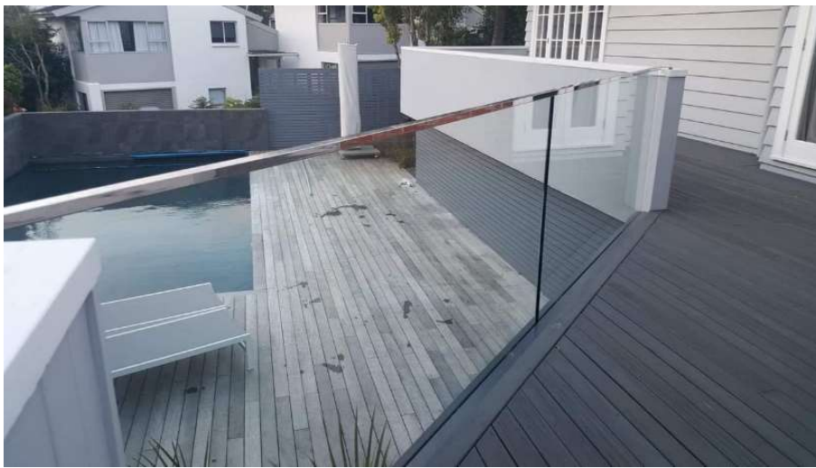
Figure 1: Photo of balcony balustrade
