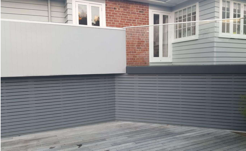
Figure 3: lower wall and balustrade junction
