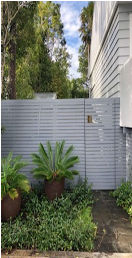
Figure 5: North gate and fence
