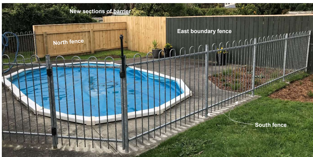
Figure 1: Photograph of the pool area and barrier
