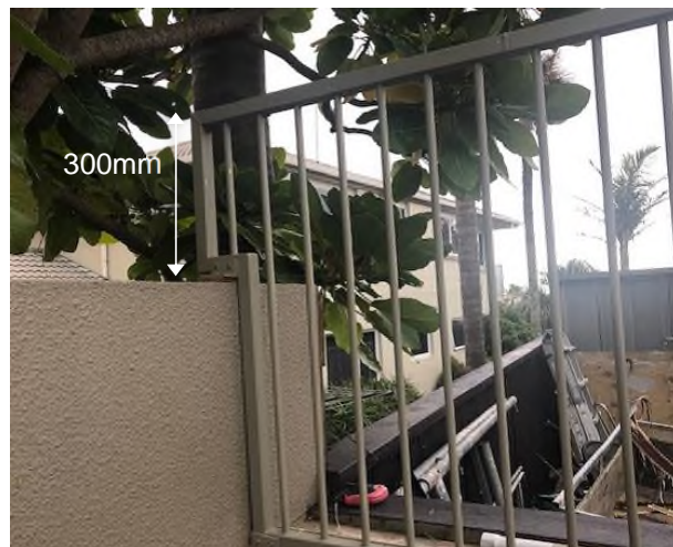
Figure 3(c): Northwest corner detail
