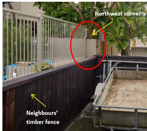
Figure 3(e): Northwest corner, seen from neighbours' property
