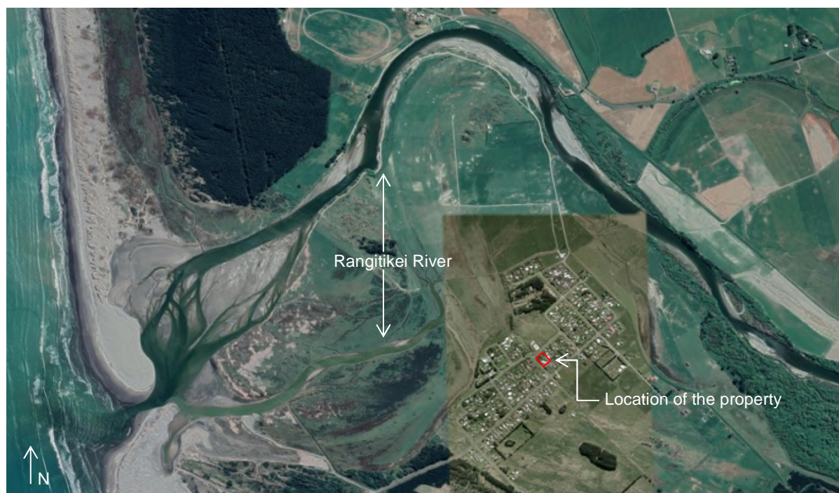
Figure 1: Aerial photograph of site (not to scale)
