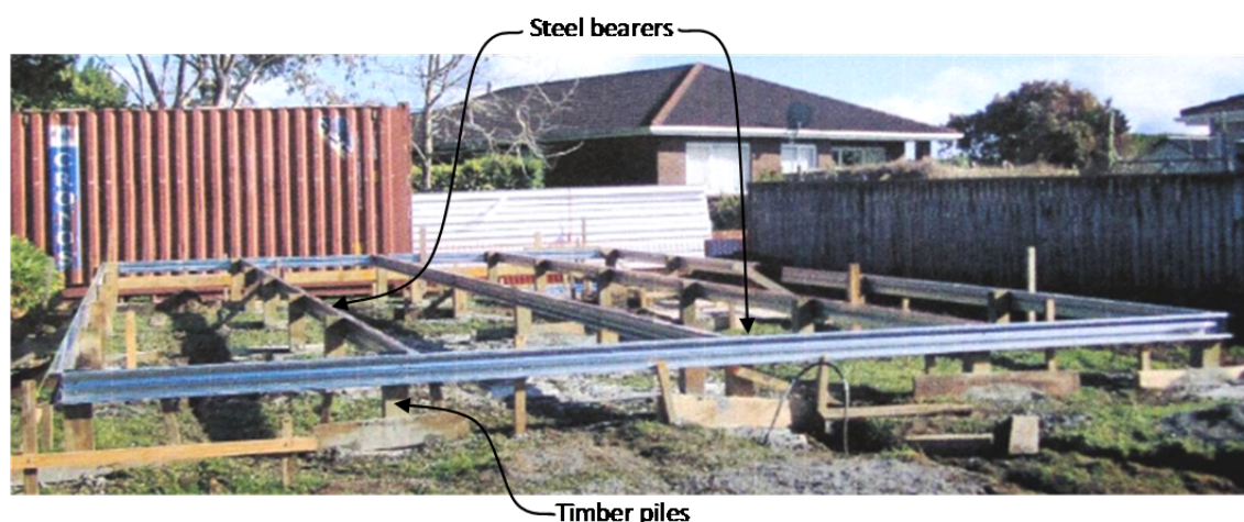
Figure 2: Typical sub-floor construction for all four buildings
