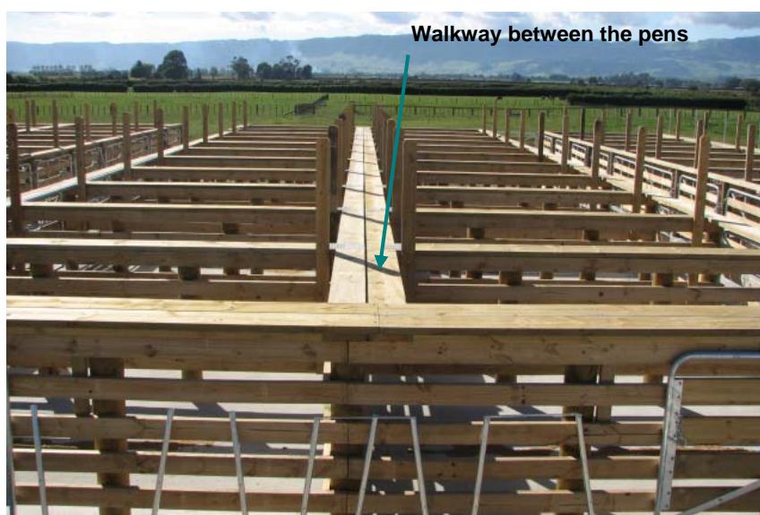
Figure 2: Walkway between the pens
