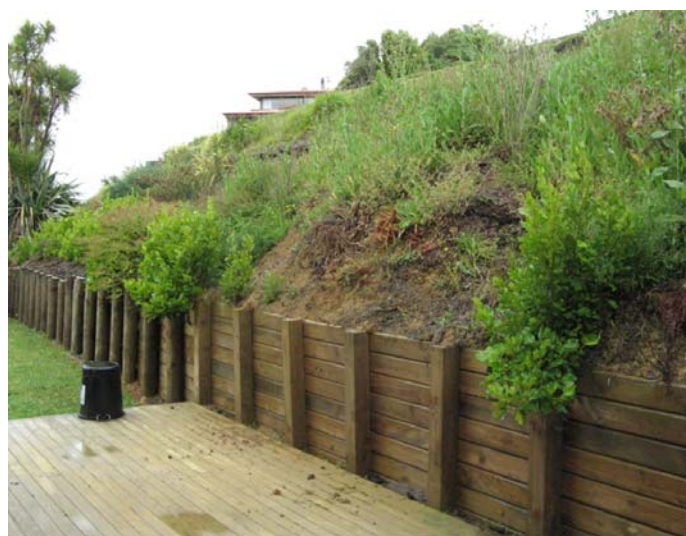
Figure 1: The retaining wall (adjacent the May 2006 landslip) as at December 2007
