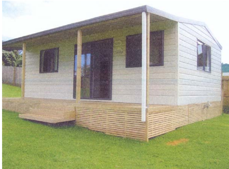
Figure 2: A unit in its final position
