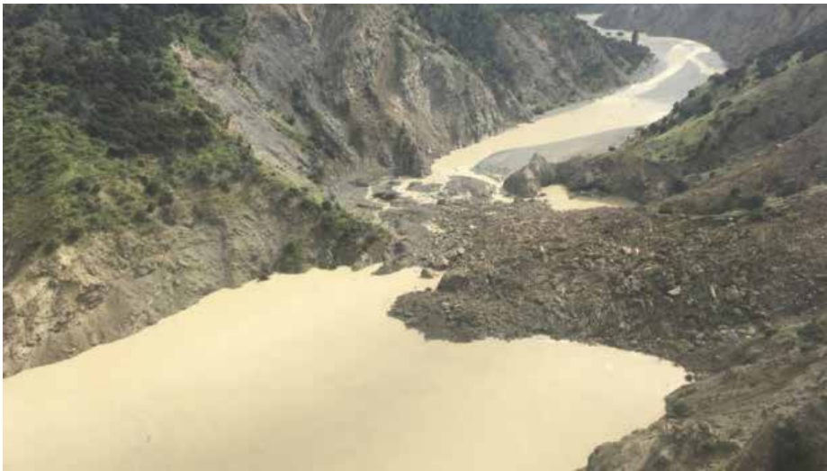
Figure 12: Landslide dam in the Clarence River, north of Kaikoūra, November 2016
