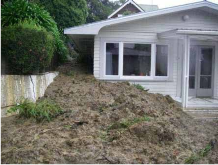
Figure 10: Impact of debris flows on a property after the 2011 Nelson storm. Credit: Tonkin & Taylor, 2011
