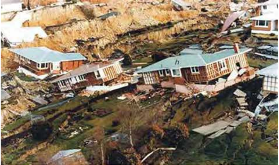
Figure 5: An example of the impact landslides can have in residential areas. Abbotsford, Dunedin, 1978
