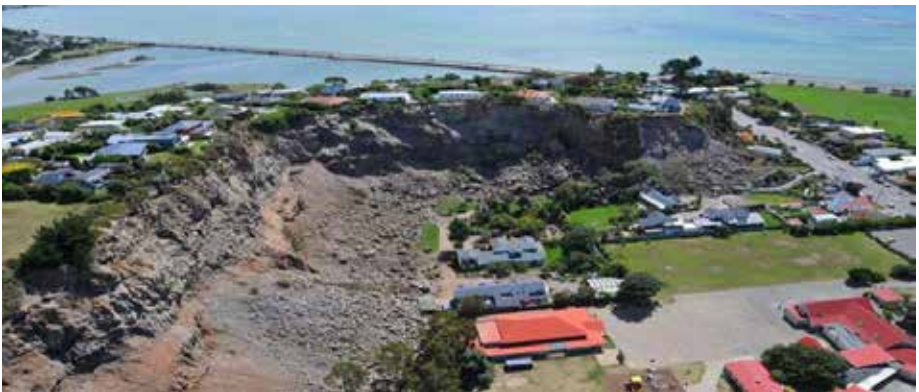
Figure 9: Cliff collapse in Redcliffs, Christchurch during the 2010–2011 Christchurch earthquake sequence
