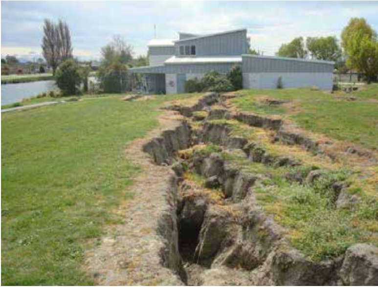
Figure 14: Lateral spreading adjacent to the Avon River, Christchurch
