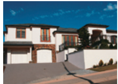
Two storey (SH) residential dwelling with an E2/AS1 risk score of 11 (deck not over living area)
