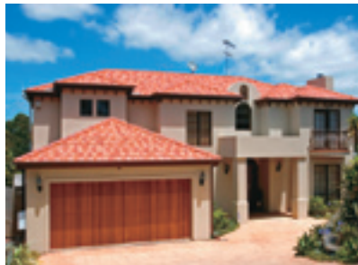
Two storey (SH) residential dwelling with an E2/AS1 risk score of 12
