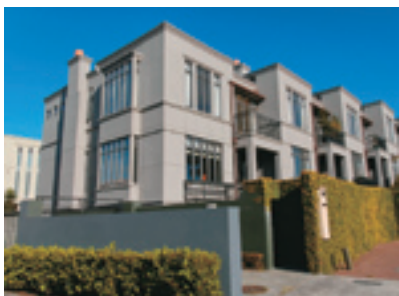
Two storey (SR) residential dwelling with an E2/AS1 risk score of 17 (vertical plane fire separation only)
