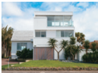
Three storey (SH) residential dwelling with an E2/AS1 risk score of 19
