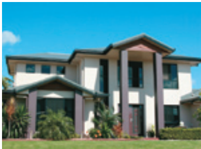
Two storey (SH) residential dwelling with an E2/AS1 risk score of 9
