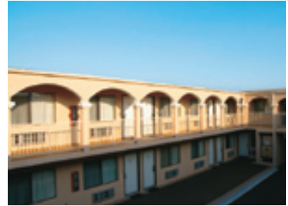
Two storey motel with less than 100 occupants
