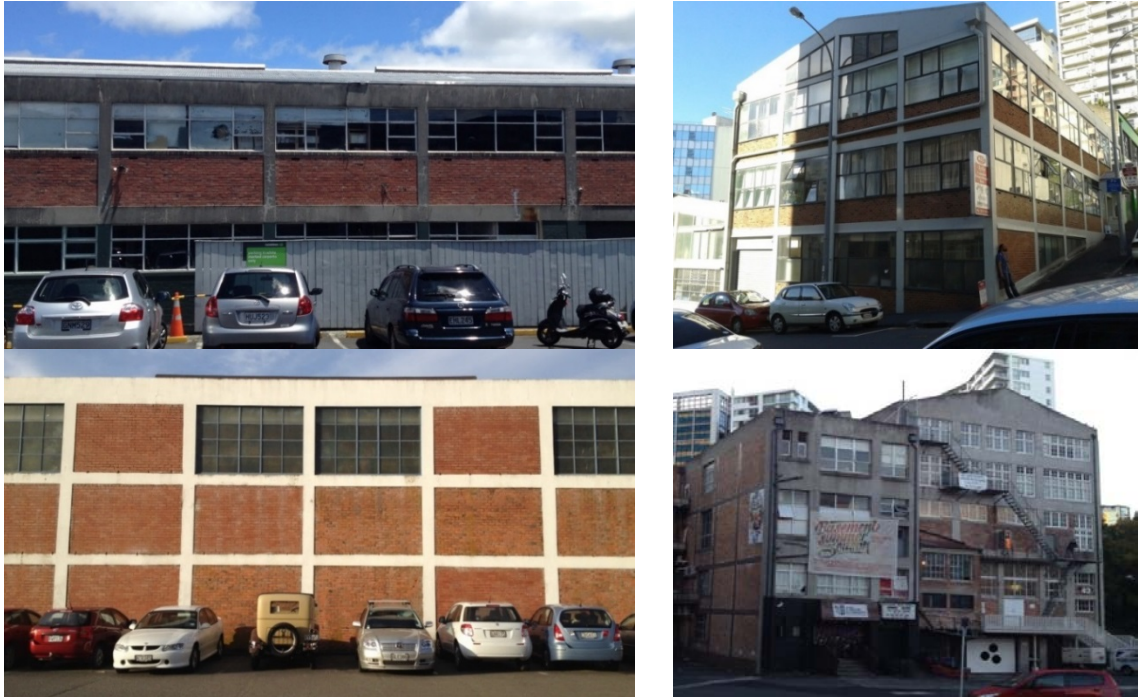
Figure C7.1: Examples of reinforced concrete frames with clay brick masonry infill (Kevin Walsh and Laura Putri)
