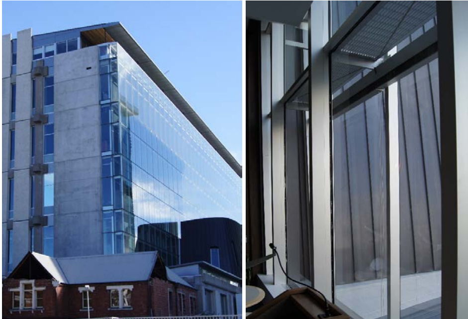
Figure C10.7: Double skin curtain wall system
