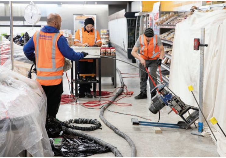
Figure 14: Installing injection tubes, injecting resin inside a supermarket
