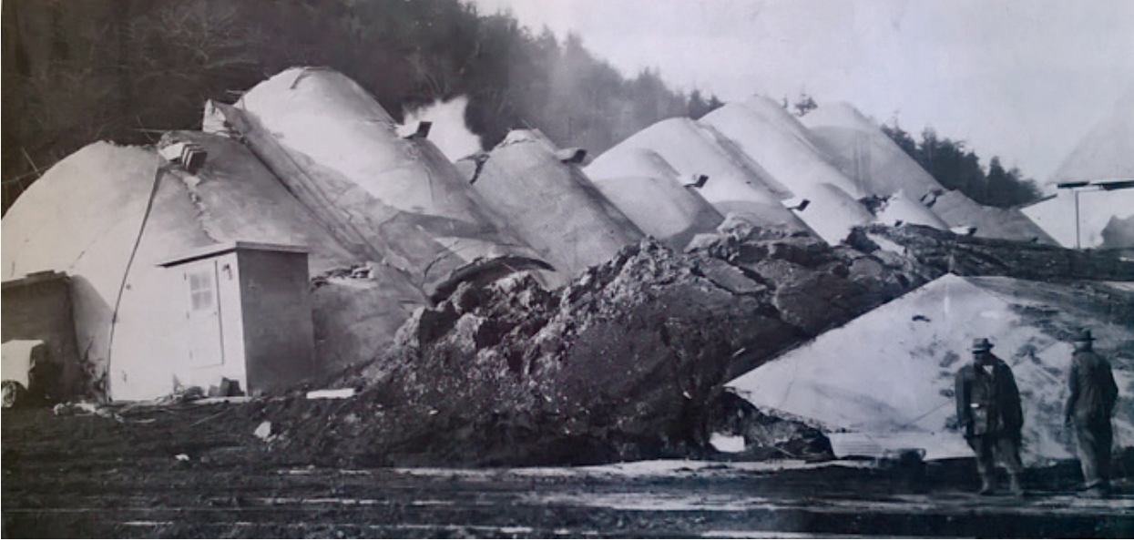
Figure 5.2: Bearing capacity failure of a silo foundation [Source: Tschebotarioff, 1951]
